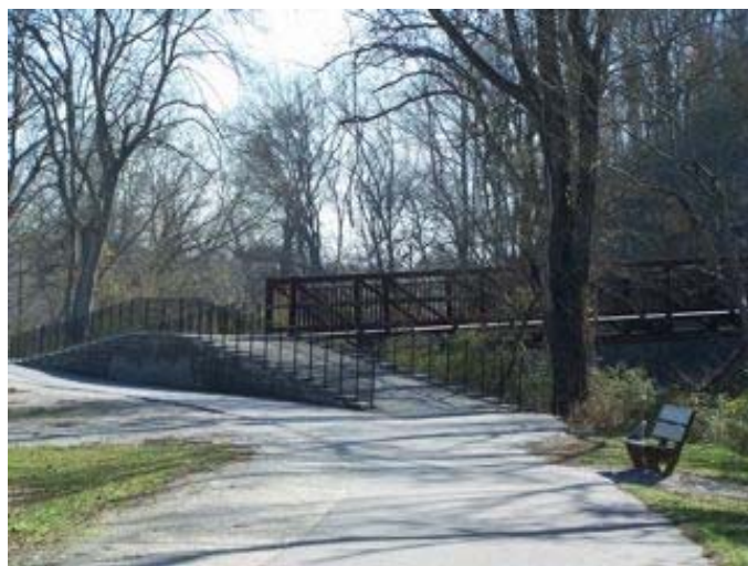
Pardue Crossing over Yadkin River to Wilkesboro
