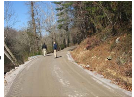
Jefferson Turnpike Greenway Trail
