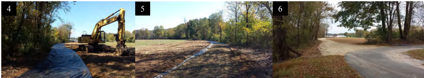
Geo-fabric installation
