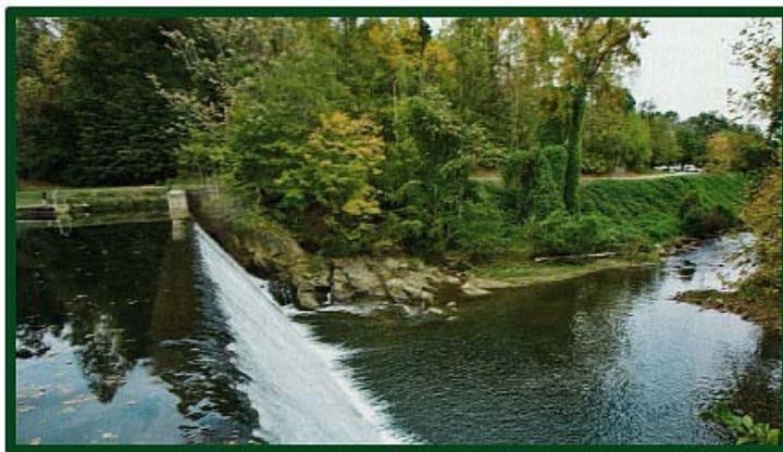
Reddies River Greenway @ spillway as seen in Southern Living
